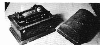
EDISON STANDARD , two-minute, oak cabinet original poor finish on top, average on base. No crank, no horn, no drive belt, otherwise complete. May operate with a new drive belt.
